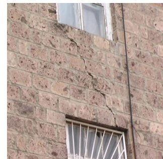
Figure 1: General view of the 4-story old damaged stone building of the school #68 to be retrofitted by base isolation and strengthened by the R/C jackets (a) and fragments of its damaged parts within the limits of the first (b) and upper floors (c)
