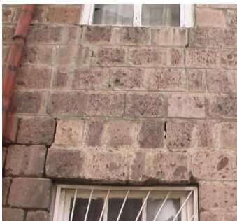
Figure 1: General view of the 4-story old damaged stone building of the school #68 to be retrofitted by base isolation and strengthened by the R/C jackets (a) and fragments of its damaged parts within the limits of the first (b) and upper floors (c)
