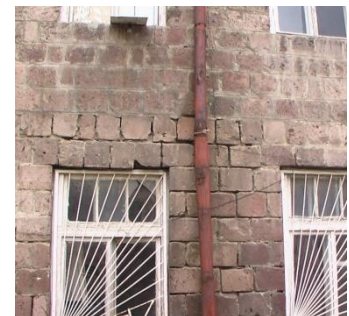
Figure 1: General view of the 4-story old damaged stone building of the school #68 to be retrofitted by base isolation and strengthened by the R/C jackets (a) and fragments of its damaged parts within the limits of the first (b) and upper floors (c)
