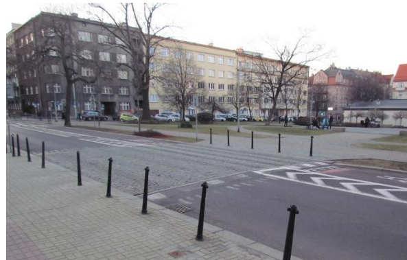
b) Marking at the beginning of the “Tempo 30” zone (Jagiellońska Street, Katowice)
