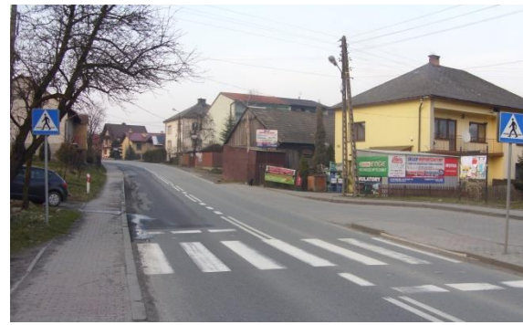
Fig. 5. A pedestrian crossing (labelled '16' on the map in Fig. 2) is an example of an unsafe crossing, as it leads to a bus stop separation island, without any additional safety features
