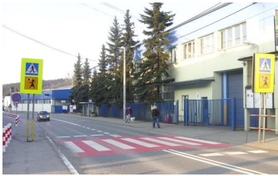
Fig. 4. A pedestrian crossing (labelled '7' on the map in Fig. 2) is an example of a safe crossing due to enhanced horizontal and vertical markings
