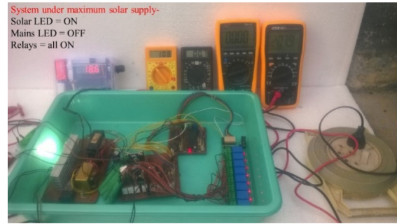
Figure 11. Hardware working under maximum solar supply.
