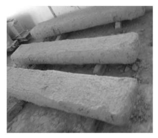
FIG. 8. BEAMS COVERED WITH SECOND LAYER OF MUD AND CHAFF
