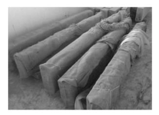
FIG. 7. BEAMS COVERED WITH GUNNY BAGS
