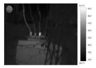
FIG. 3. THERMOGRAPH SHOWING LOAD UNBALANCE ON 200KVA TRANSFORMER LOCATED AT QASIMABAD CITY, HYDERABAD
