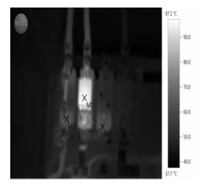
FIG. 7. THERMOGRAPH SHOWING UNBALANCED LOADING AT FUSES AT TELEPHONE EXCHANGE HYDERABAD
