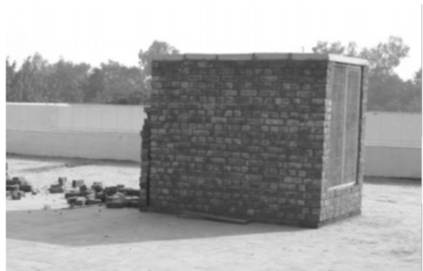
FIG. 3. PHOTOGRAPH OF THE TEST MODULE
