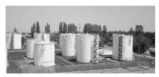
Figure 1 – Oil tanks type RVS (RVS-5000, RVS-3000)
