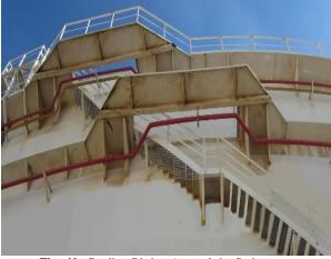
**Fig. 40:** Cooling Piping Around the Stairway 9-Pressure Gauge: it is required by NFPA 15 to install a pressure gauge at the location of the most remote nozzle [16]. The gauge gives the status of the system and its operability. This requirement is not observed in most cases.
