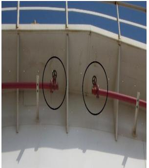
Fig. 38: Ring Main with a Valve at the End
