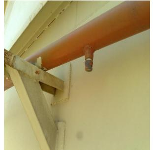
Fig. 29: Water Spray Nozzles Installed in 6 O'clock Position of Ring Main
