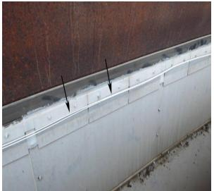
Fig. 57: Linear Heat Detector
