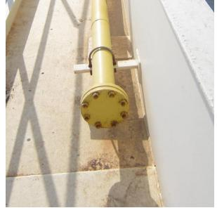
**Fig. 60:** Foam Ring Main with Flanged End 12-Foam System for Fixed Roof Tanks: use of ring main for distribution of foam solution to foam chambers for protection of fixed roof tanks containing flammable liquids [12] is not allowed
