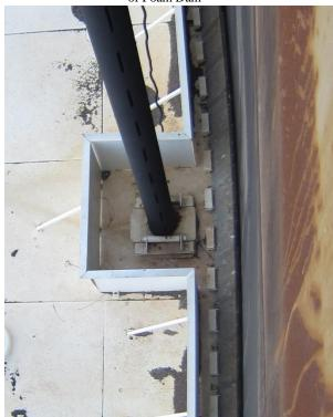
Fig. 12: Good Design of Foam Dam around Guide Pole
