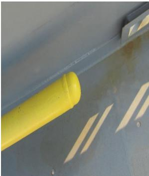
Fig. 59: Foam Ring Main with End Cap
