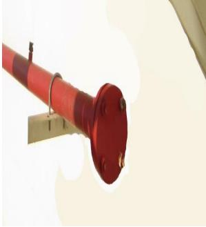
Fig. 37: Ring Main with Flanged End
