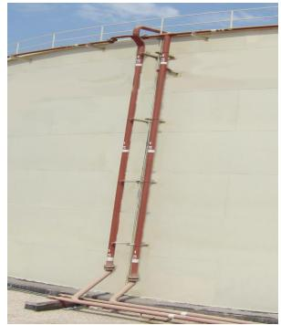
Fig. 35: Separeated Roof and Shell Water Spray Cooling System
