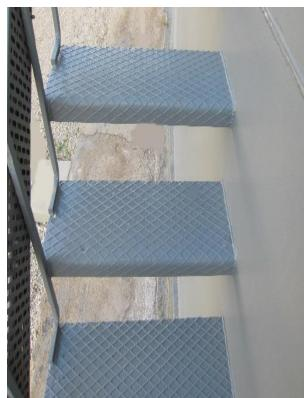
Fig. 17: Spiral Stairway with Steps Attached to Tank Shell
