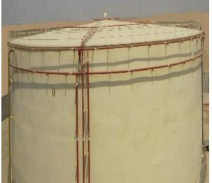
Fig 33: Cooling System for Shell and Roof of a Fixed Roof Tank
