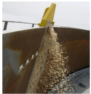
Fig. 43: Throwing of Foam Stream by Foam Pourer
