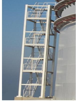
Fig 18: Staircase Structure Constructed Next to Tank
