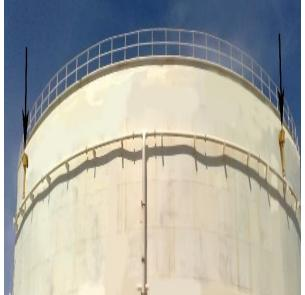
Fig. 61: Installation of Foam Chamber on a Header for a Tank Containing Flammable Liquid
