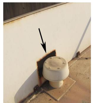
Fig. 5: Detrimental Foam Dam Modifications
