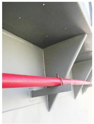
Fig. 13: Water Curtain Blockage by Triangular Support Members
