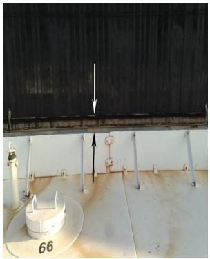
Fig. 9: Inappropriate Foam Dam Height
