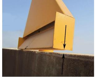
Fig. 46: Foam Pourer Not Fixed to Top Angle
