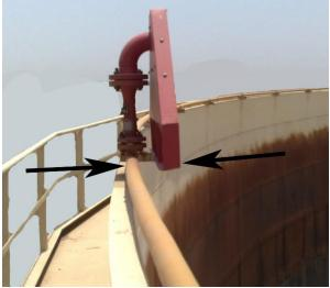
Fig. 49: Foam Pourer Sticking inside the Tank
