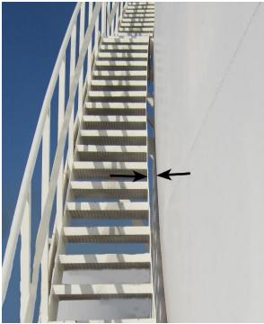
Fig. 20: Spiral Stairway Separated from Tank Shell PROBLEMS ASSOCIATED WITH THE COOLING SYSTEM
