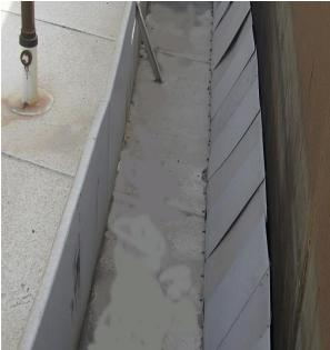
**Fig. 10:** Inappropriate Foam Dam Width 5-Foam Blockage inside Dammed Area: foam dam design around guide and anti-rotation poles and other tank components located in or near rim seal area is important because of the need for flow of foam within rim seal area between two adjacent discharge devices. In some tanks, the foam dam is so designed
