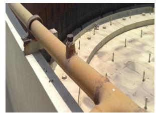
Fig. 56: Tap for Pressure Gauge
