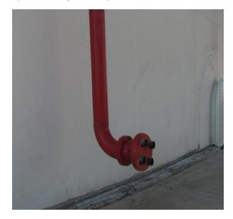
Fig. 21: Piping Terminated at Tank Bottom
