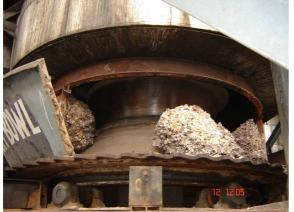
Figure 1: Ash bowl arrangement with guide roller
