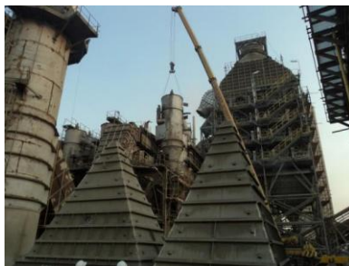
Fig.22: Demolishing of the Gravel Bed Filter.
