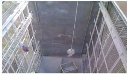
Fig.9: Step No.2-Strip off the ESP Internals.
