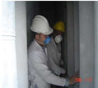
Fig.13: Adjusting filter bags.
