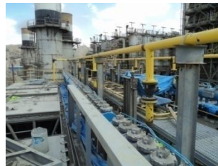
Fig.11: Installing new gas plenum.
