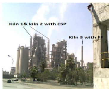
Fig.14: Comparison between ESP stacks and converted ESP into FF stack in Assiut Cement Company.
