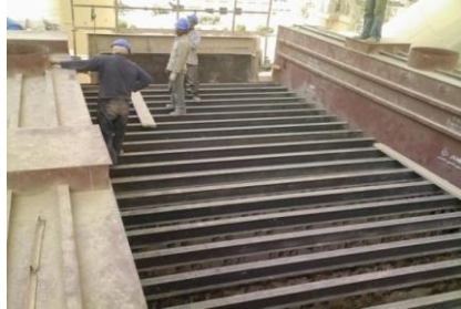
Fig.8: Step No.1-Cut the ESP roof.
