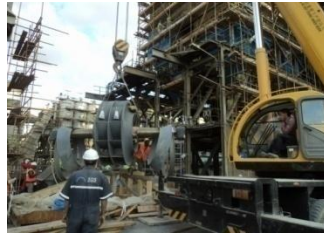
Fig.12: Replacing old ID fan.
