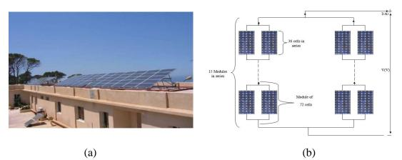
Figure 3. (a) Installation of the photovoltaic generator on the roof of CDER, (b) diagram of each generator.
