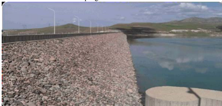
Fig. 1: Upstream slope of Alavian reservoir dam
