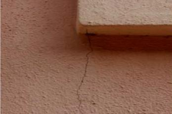
Figure 3: Crack between bay window corners
