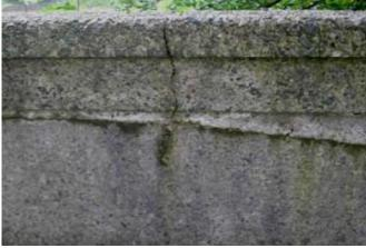
Figure 2: Cracks at the centre of panel
