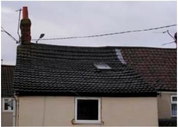
Figure 10: Sagging of roof
