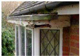
Figure 7: Timber decay of Flat roof
