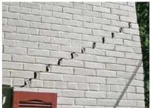
Figure 1: Foundation wall cracks
