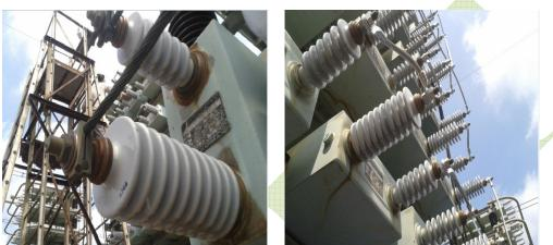
Fig 1.2 Filter capacitor bank without Lug Fig 1.3 Filter capacitor bank with Lug
