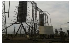
Fig. 1.4 Bird fault frequently occurs on this filter banks
