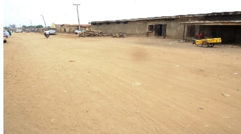
Plate 2: Bauchi Street earth road without side drainage in a minor road.
