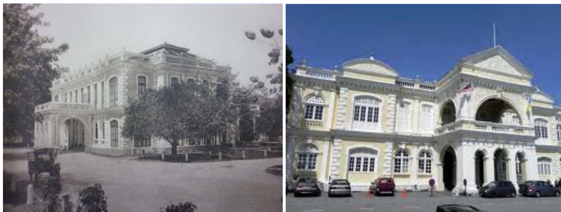
Figure 1: Penang Old Town Hall in 1900s (left) and Penang Old Town Hall in 2012 (right)
