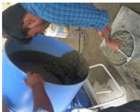
Fig. 4 Fresh concrete mix
