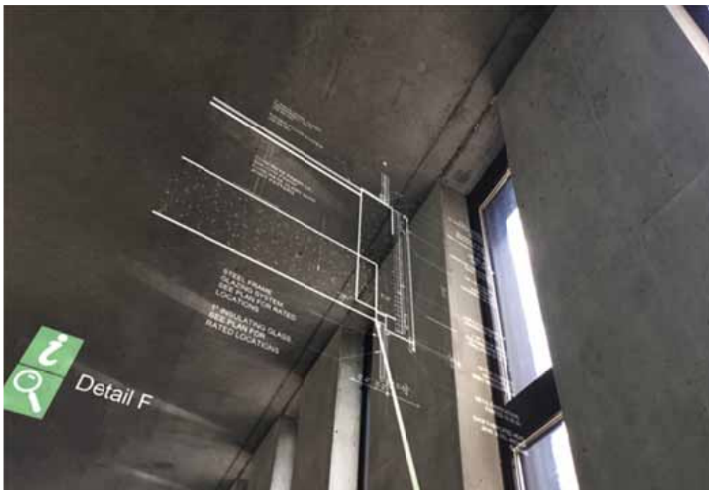
Figure 9. In-situ roof-wall detail with associated icons
