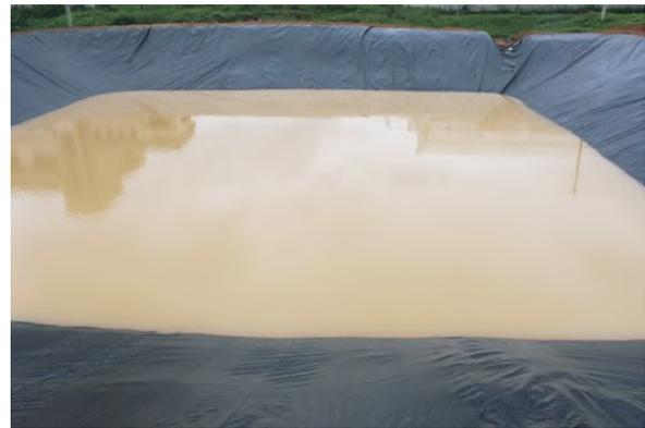
Fig. 1 : Plastic lined water harvesting pond.
