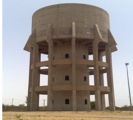
Figure 3: Storage Tower of MWTP
