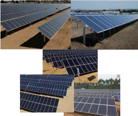
**Figure 2.** Examples for single line and double lines of PV modules per row
