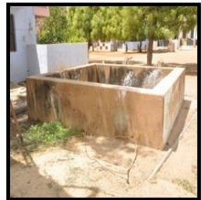
Station III (Church open well)
