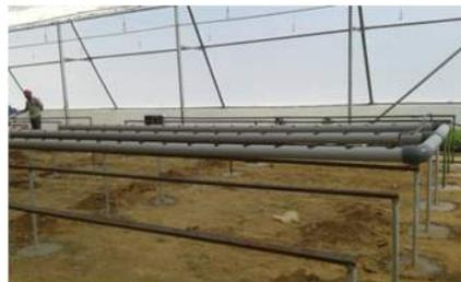
Fig. 1 : PVC pipes of 4 inch diameter with 6 m length each was placed on 27 Iron angle rods.
