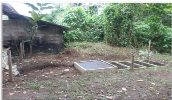
Figure 5. Biogas technology project in Malvar
