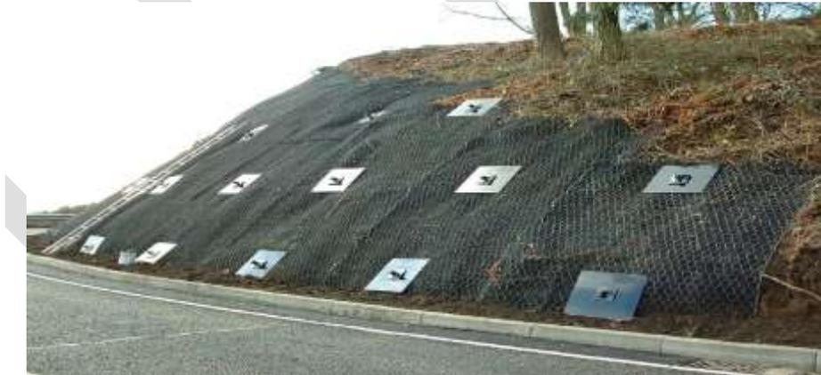
**Figure 2:** Actual picture of soil nailing in hill slope
