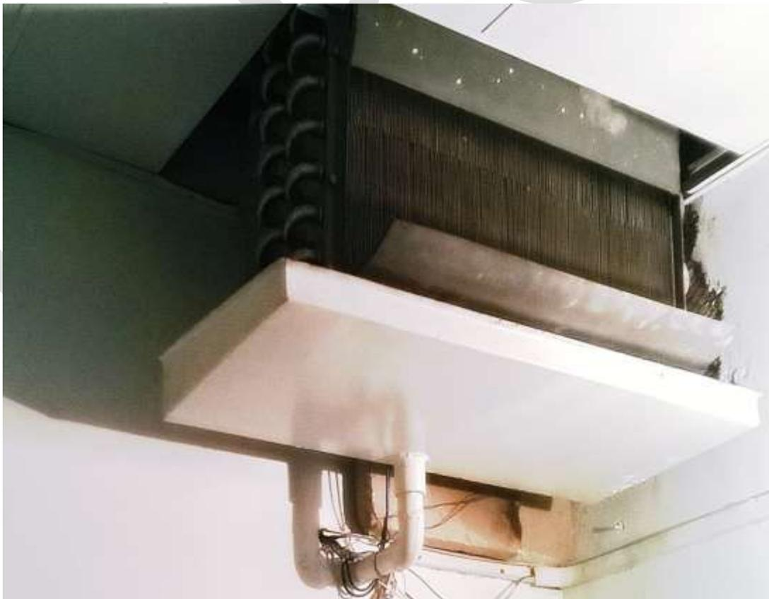
**Figure 2** Ceiling Mounted Cooling Coil inside Cold Chamber
