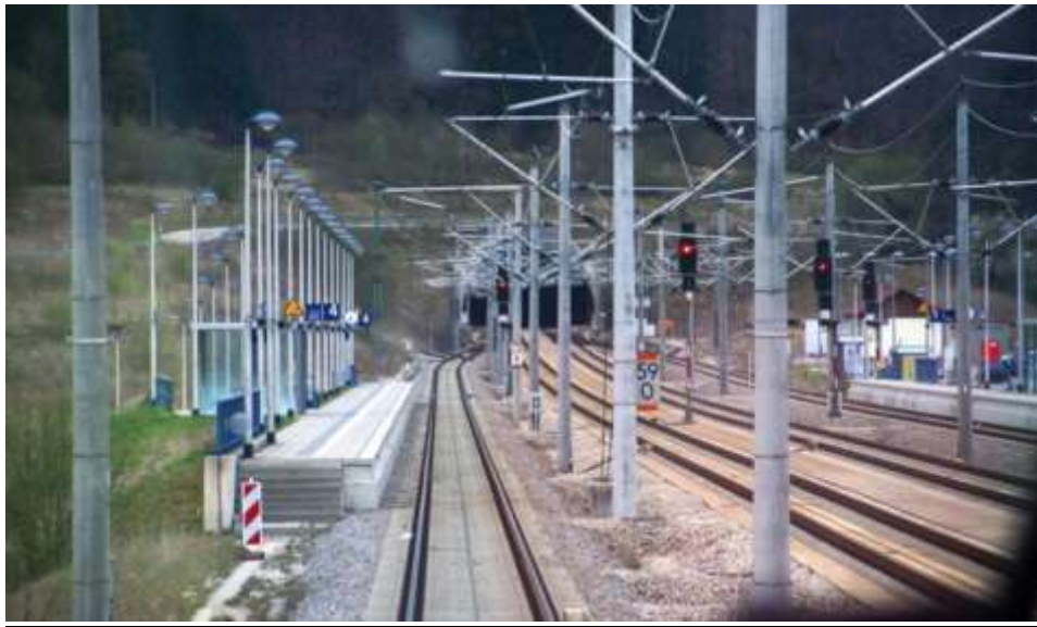
Fig. 14. Kinding station on high-speed line Nuremberg-Ingolstadt [3]
