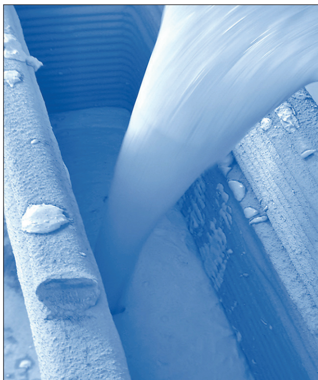
Fig. 4. Filling with foam gypsum nanocomposition of vertical enclosing 3D constructions
