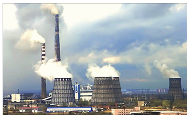
Fig. 3. External view of the city CPP
