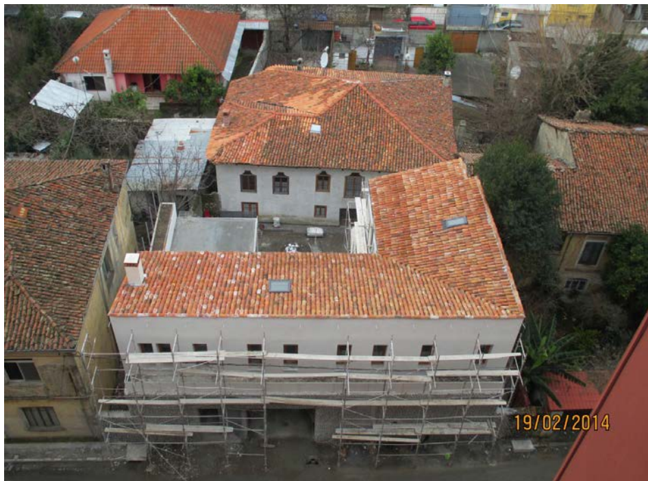
Figure 3. The Art House construction site, 2014.
