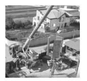
**Figure 10.** Free standing prop- turbine lifting by crane.
