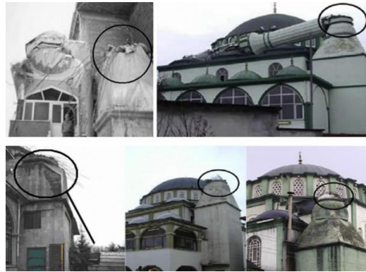
Figure 2: Failures or damaged RC minarets (Sezen et al. 2008)
