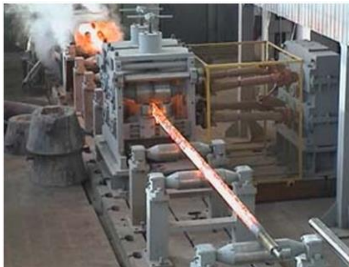
Figure 8. Horizontal continuous casting machine for steel billets with a diameter of 0.08 m designed by LLC «SPETSMASH», commissioned in 2002–2003 (press release «SPETSMASH» LLC, 2005)
