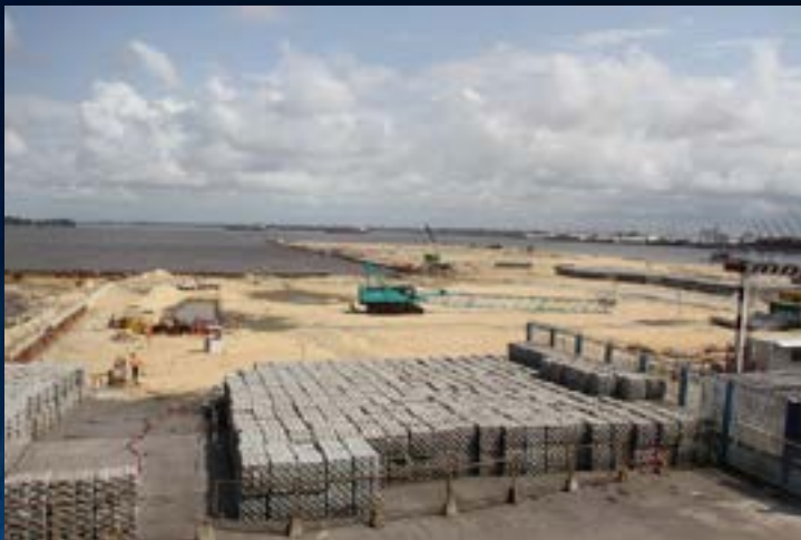
Construction of New Mineral Terminal
