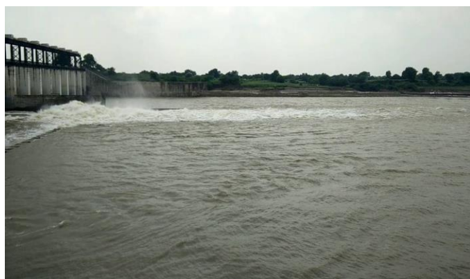
Fig. 1: Vishnupuri Dam constructed on Godavari River in Nanded
