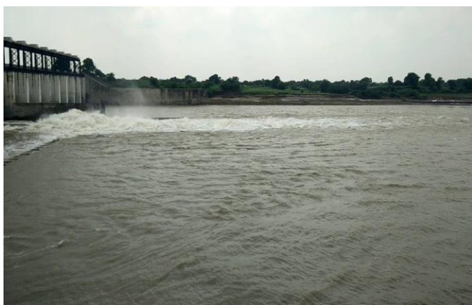
Fig. 1: Vishnupuri Dam constructed on Godavari River in Nanded
