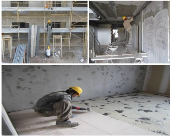
Fig. 1: Some jobs of construction industry involved in ergonomic risk factor assessment process.
