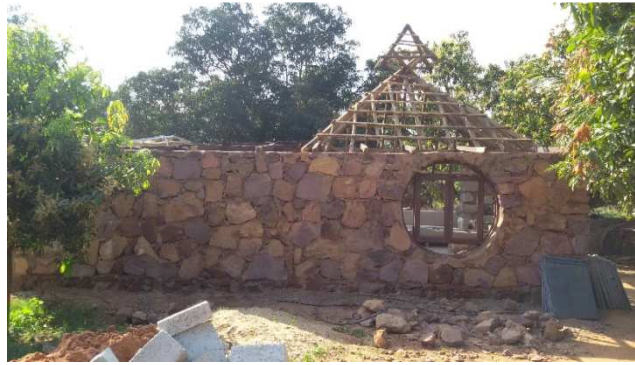
Figure 4: Palm Trunk Roof Frames and Laterite Stone Wall
