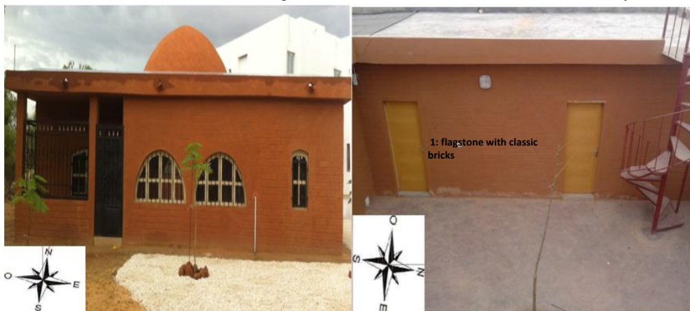
Figure 2: geo-concrete building-test in Polytechnic School of Thies
