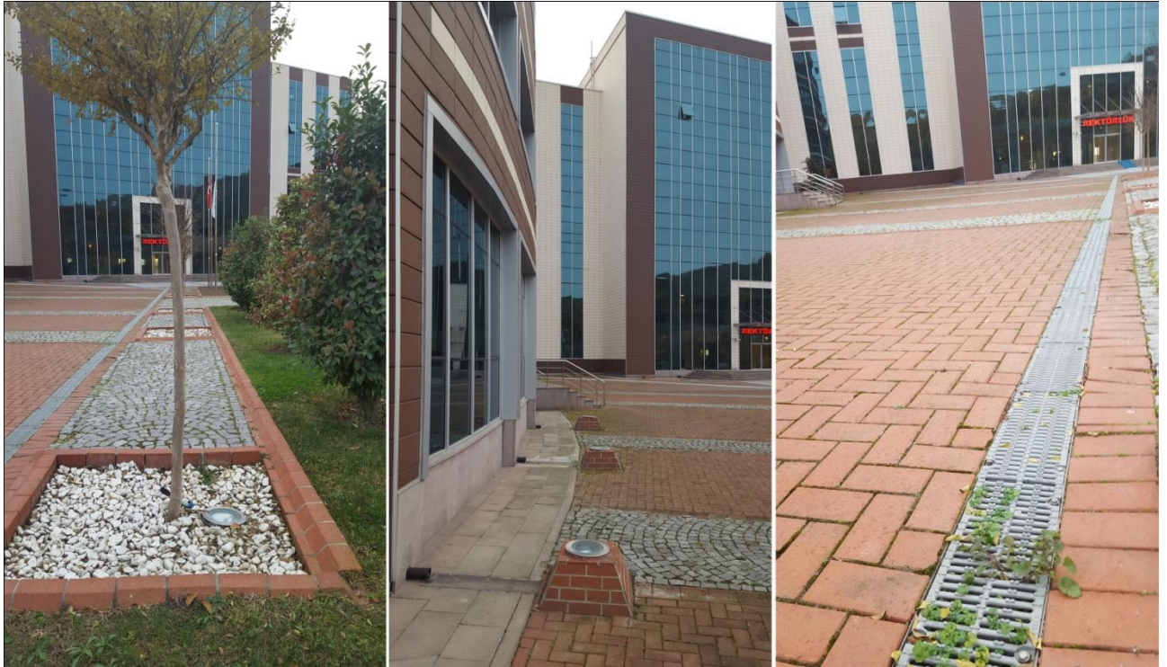
Figure 11: Lightening elements and the drainage canal
