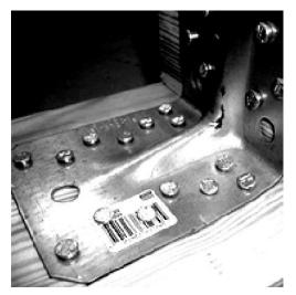
**Fig. 6.** Example of the fixing of carpentry joints in the timber – timber combination – the proper nails placement [8]
