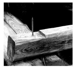
Fig. 5. The broken connection with rafter nail [8]
