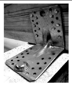
**Fig. 9.** Example of fixing of carpentry joints, a timber – concrete combination – the failure because of too large distance of a bolt to the break line [8]
