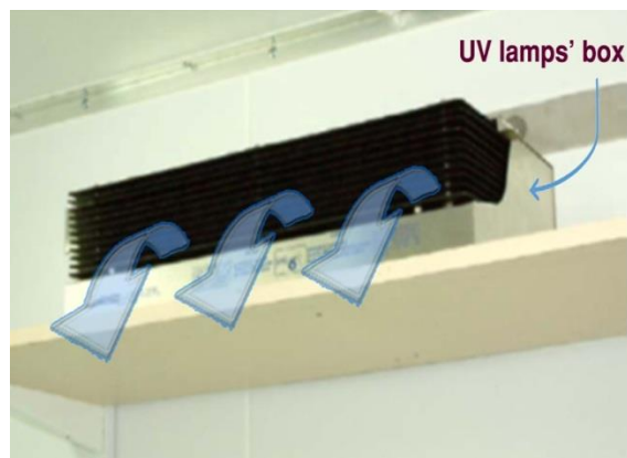
Fig. 3: A schematic of UV system for upper air of the room Photocatalyst
