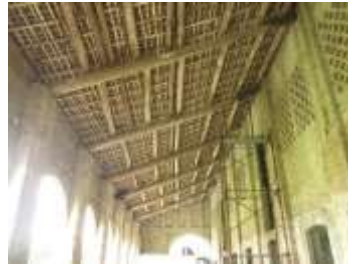
Figure 25. Lateral aisles: a) masonry wall, b) the wooden roof structure.
