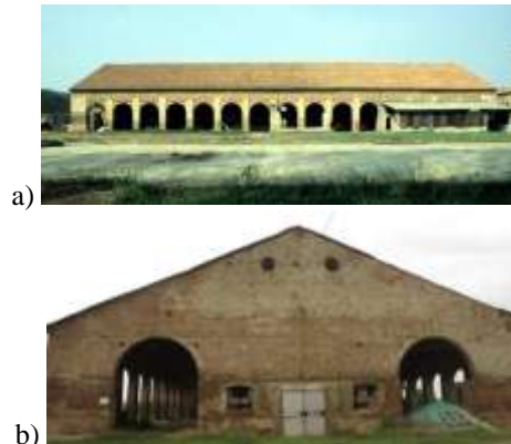
Figure 21. Bugno Martino (MN) old barn: (a) north elevation, (b) west elevation
