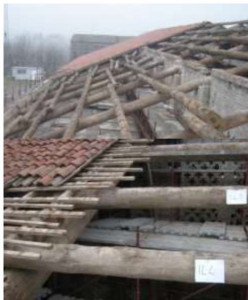
Figure 26. Flexible timber roof of the barn.
