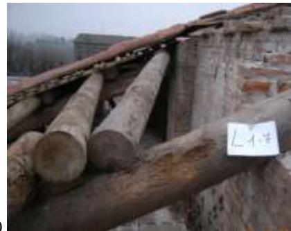
Figure 34. a, b) Damages in joints of the wooden truss; c) absence of connectors between wood rafters and secondary beams
