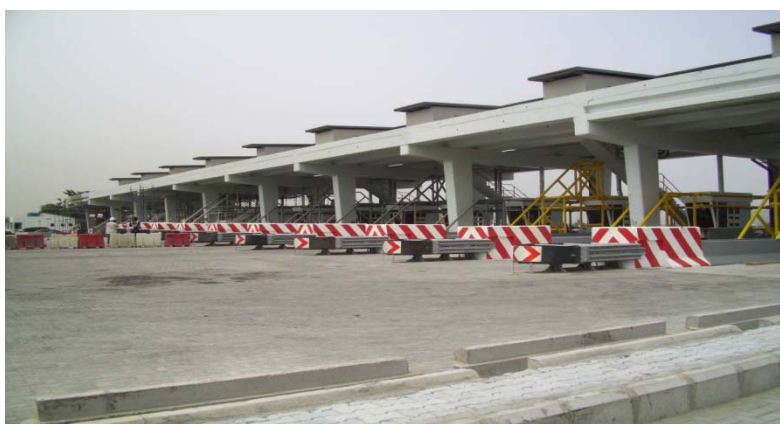
Figure 2 Admiralty Toll Plaza – Completed
