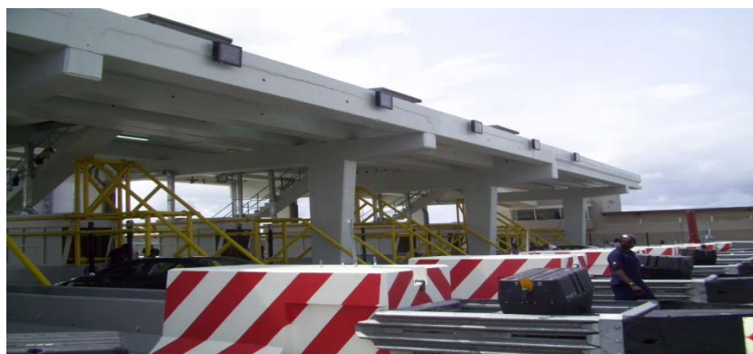
Figure 3 Conservation Toll Plaza - Completed
