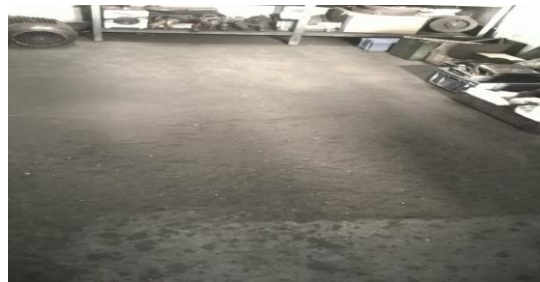
Fig 22 Floor of maintenance dept. (After)
