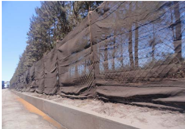
Figure 5 Wind fence (photo of the author's field visit)
