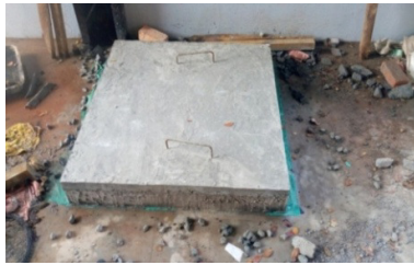
Fig. 3 Slab with SFRC topping
