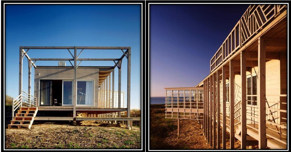
Figure 7 & 8: Inside out balloon structure of the house,
