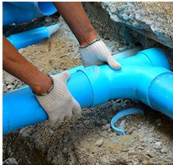
**Easy to Install and Maintain:** plastics can be installed easily with less requirements of management and impenetrable. They are light in weight and their flexibility enables the possibility of soil movements in plastic pipes.
